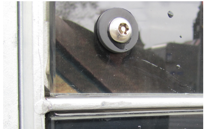
3. Detail, Amsterdam Centraal Station.
