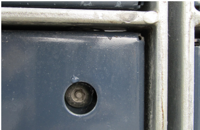
2. Detail, Amsterdam Centraal Station.
