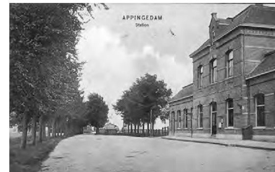
4 Station Appingedam, geopend 15 juni 1884, foto 1900
